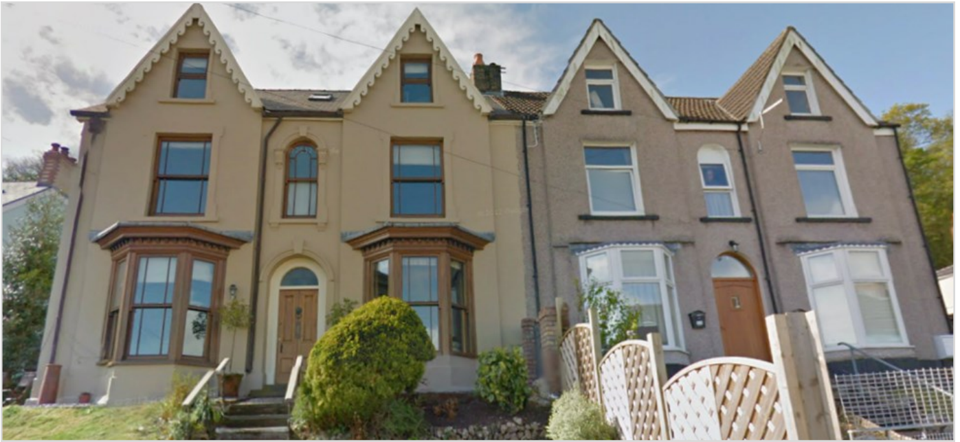
Example of a late Victorian grouping where property on the right has lost some of its heritage detail – fenestration, decorated bargeboards and ground floor bay window surround
