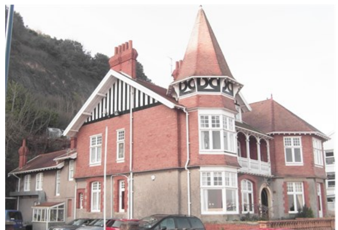
Bristol Channel Yacht Club, a listed building located along Mumbles Road
