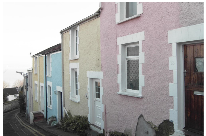
Coordinated renovations and painting schemes for a traditional terrace would have been improved with the retention of appropriate heritage designs of fenestration and doors. The widespread use of uPVC throughout the Mumbles Conservation Area is not the preferred option, but where uPVC requires less maintenance because of the impact of the sea air, it will be important that appropriate traditional designs of windows and window bars are used with the necessary reveals.
