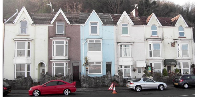
This attractive sea front terrace of Victorian houses displays the concerns of gradual change: loss of chimney stacks and pots; replaced gable barge boards; the removal of the arched top floor window openings; two inaccurately rebuilt two storey bays; changed window fenestration; door openings and doors have been replaced; and the pebble-dash wall finish does not respect the traditional design.
