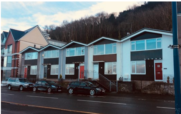
Inappropriately styled development that does not integrate with adjoining buildings can negatively impact upon the heritage townscape
