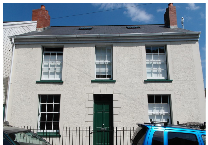
A good example of renovation of a residential dwelling on Overland Road.
